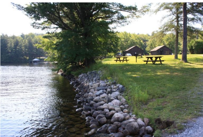
Shoreline Protection at Day Use Area
