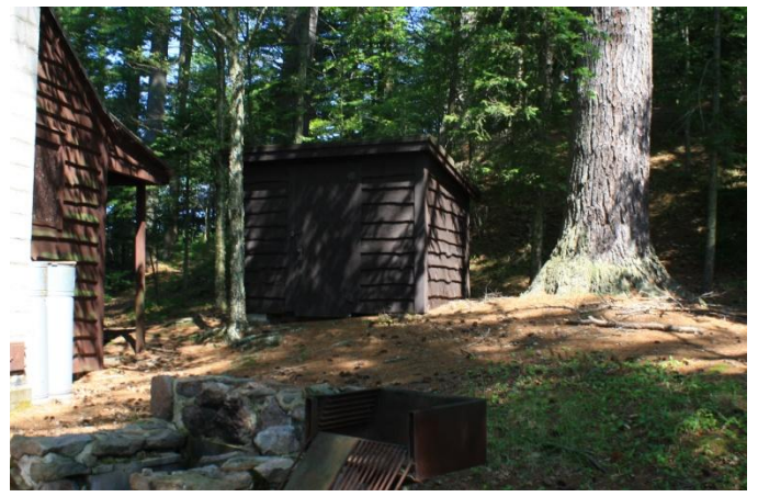
Alger Island Storage Building
