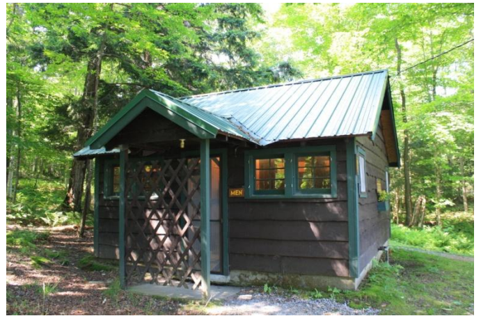
Day Use Area Comfort Station
